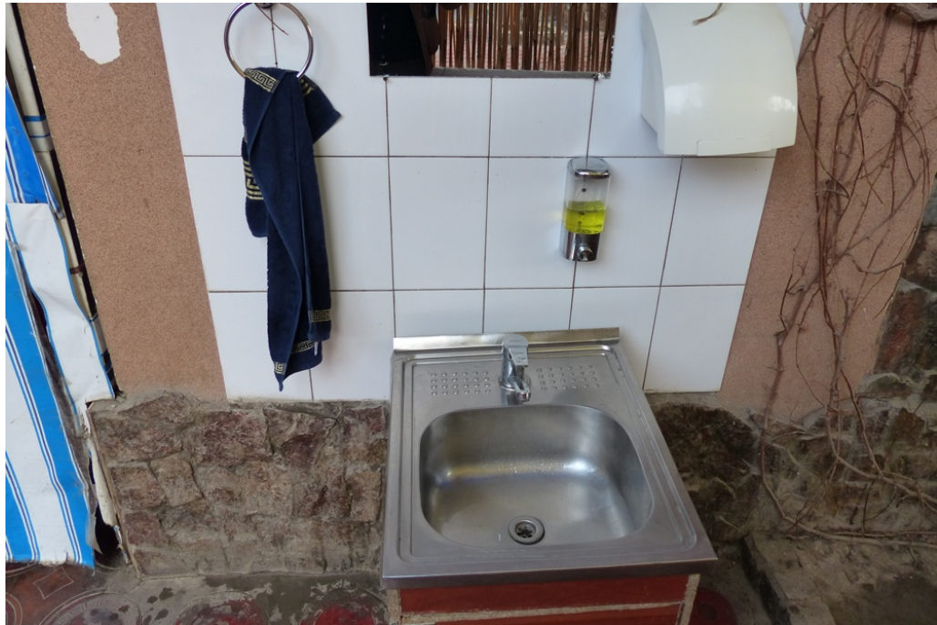
Figure 50: A proper handwashing facility, with a good quality tap, liquid soap distributor, mirror and paper.
