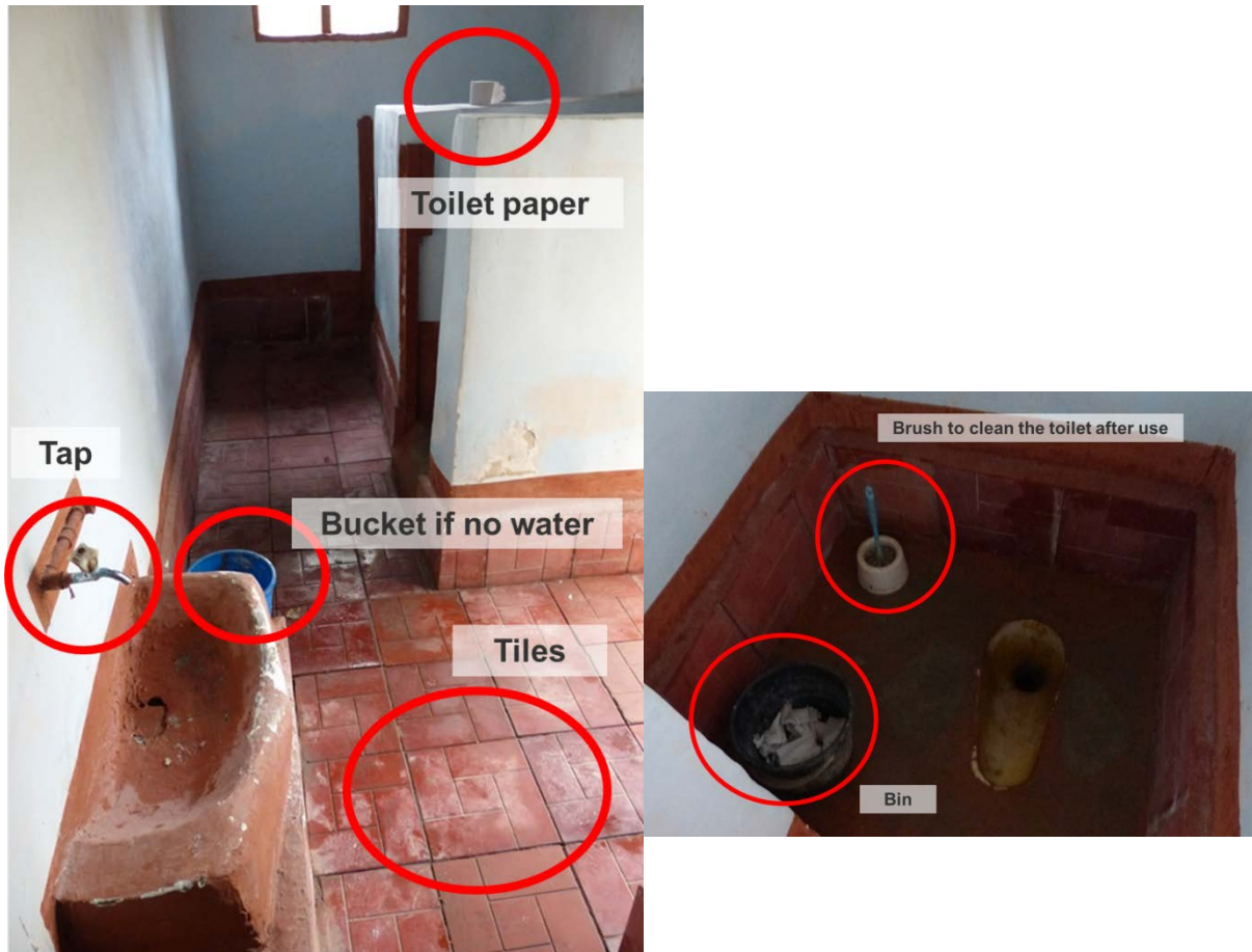
Figure 52: Good example of toilet interior design.
