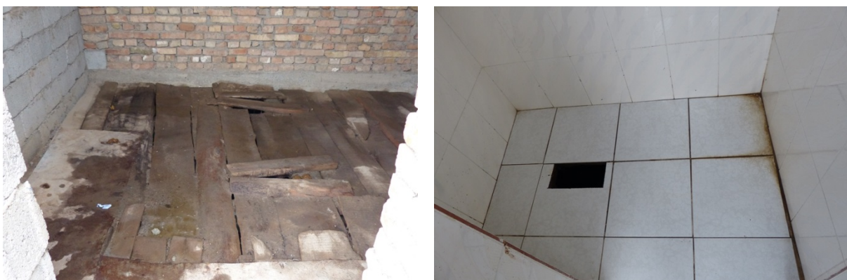
Figure 45: Two different surfaces; the ceramic surface on the right is much easier to clean and thus provides safer and more hygienic conditions.
