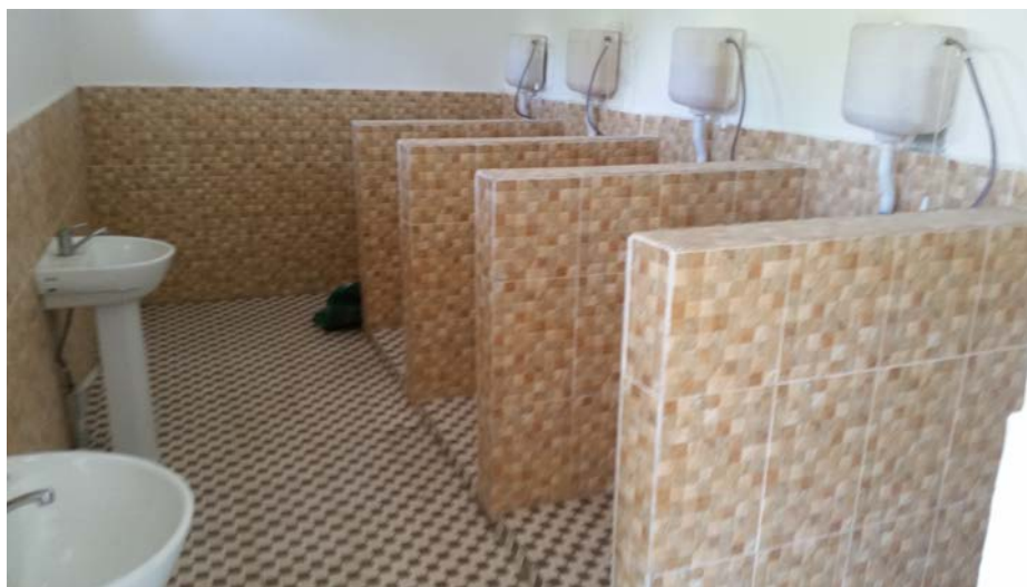
Figure 26: Students toilets, school 71, Penjikent
