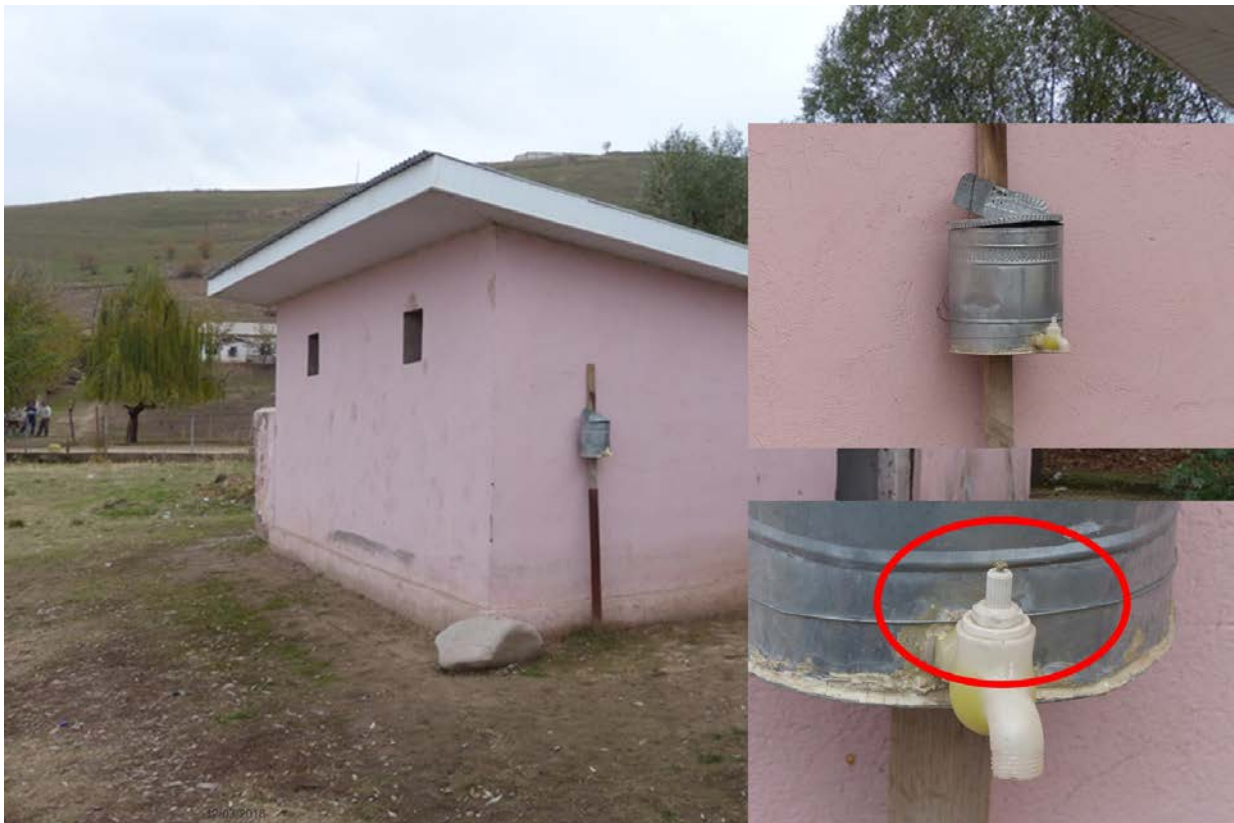
Figure 16: Typical handwashing station in schools
