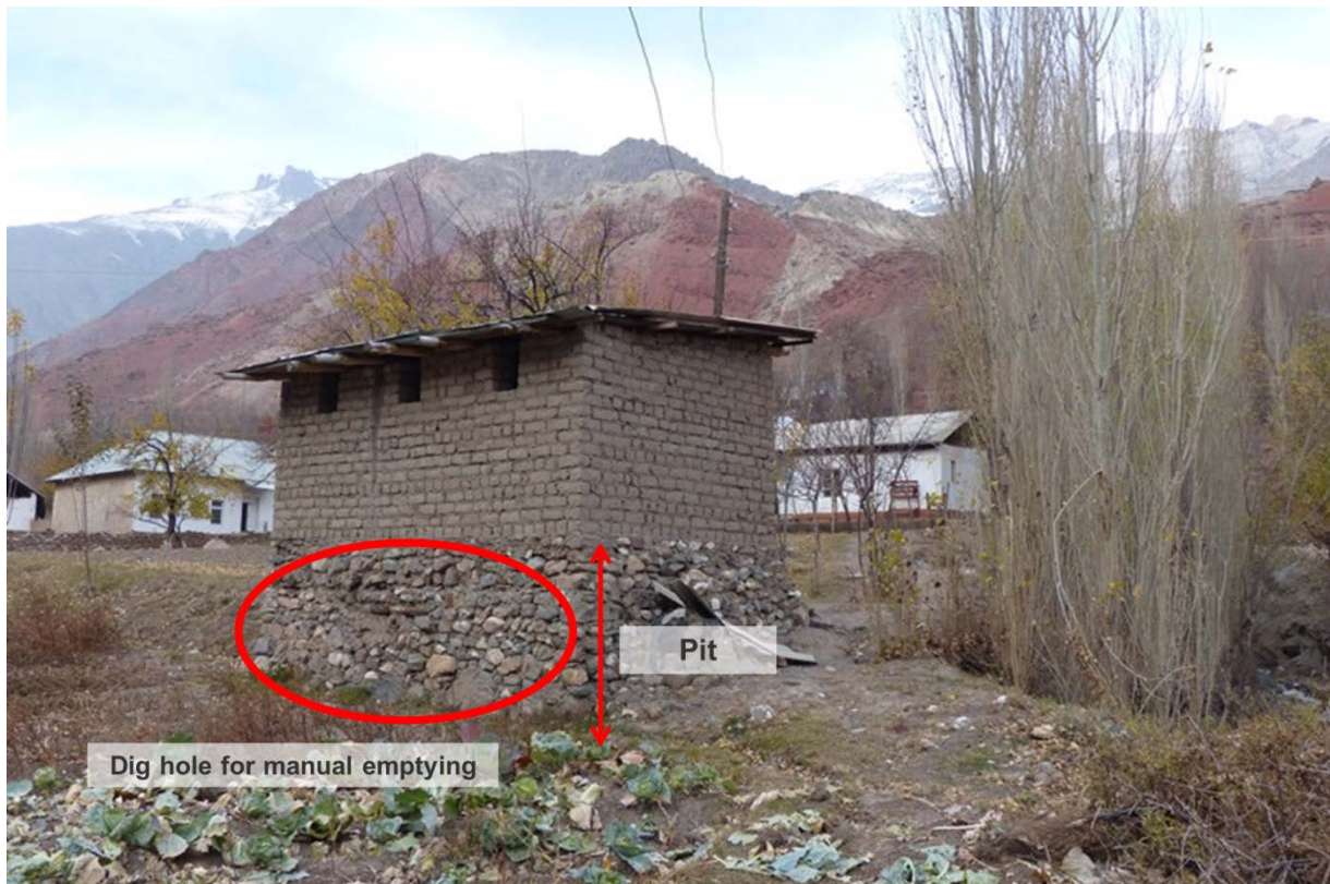
Figure 6: School toilet block in the Fann mountains (Ayni), with reuse of composted excreta in gardening
