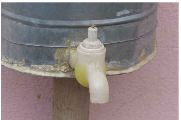
Figure 5: Typical design and maintenance issues encountered in school toilet blocks in Tajikistan
