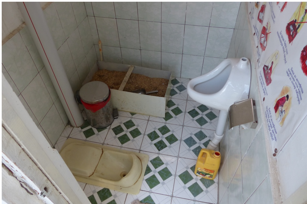
Figure 43: A urine-diverting dry toilet implemented by ISW in the Sughd region, including also a waterless urinal.
