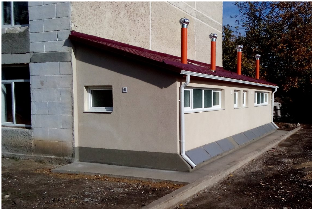
Figure 48: UDDT-based school toilet block attached to the school building in Moldova (picture: SKAT)
