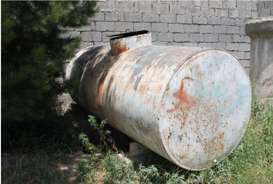
Figure 10: Example of deteriorated tank used to store water in school
