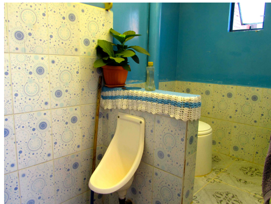
Figure 5.6: Interior of one of Sumaj Huasi's UDDTs.
