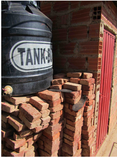
(a) 450L private water tank in the OTB Villa Montes.
