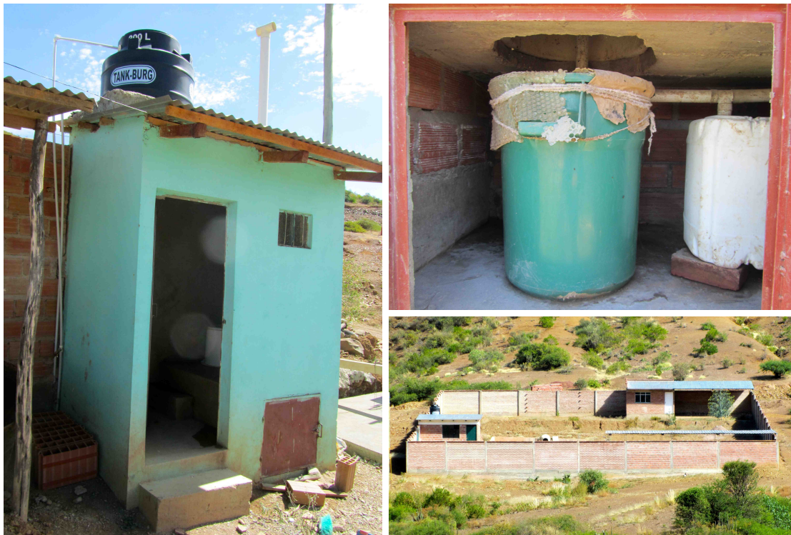
Figure 3.6: Clockwise: Exterior of a UDDTs built by ADRA, chamber for the faeces bucket and urine jerrycan, faeces treatment plant in Llave Mayu.
