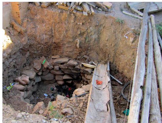
Figure 7.4: Construction of a permeable pit latrine in the OTB Florida.
