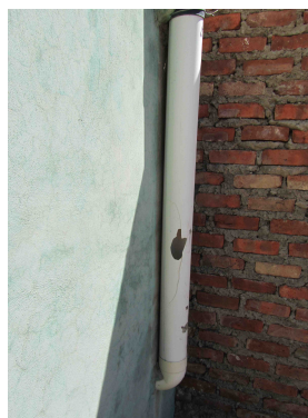
(b) Broken aeration tube
