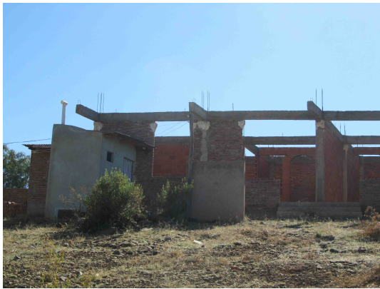
(a) UDDT next to an uncompleted house in the OTB 20 de Mayo.
