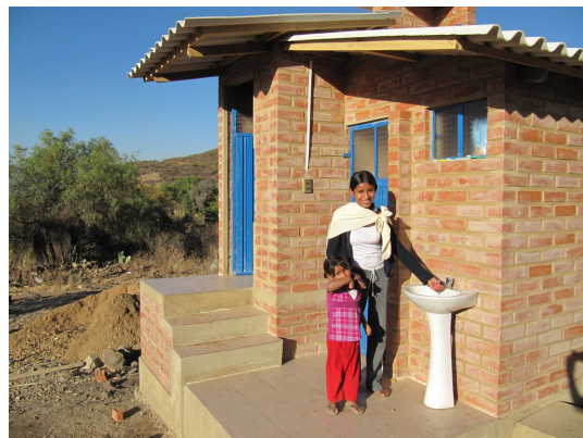
Figure 5.3: Design of the bathrooms in the OTB Higuera: UDDT (back) and shower (front), foto taken by the Fundación Aguatuya.
