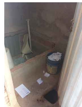
(c) UDDT transformed into simple pit latrine
