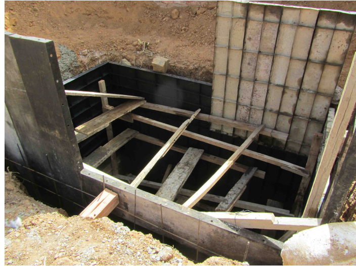
(b) Construction of a 12'000L private water tank in the OTB Llave Mayu to benefit from lower water prices.
