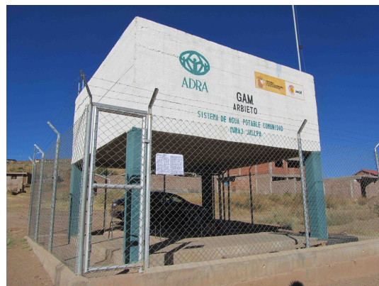
Figure 3.11: Water tank in the OTB Yuraj Jallpa (filled by water trucks).
