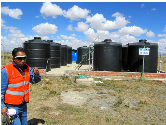
(a) 5000 L storing tanks for the urine in Sumaj Huasi's treatment plant.
