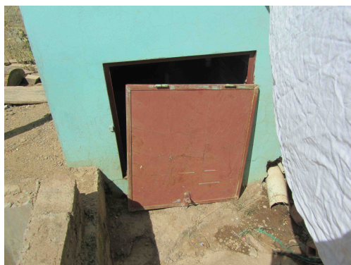
(a) Broken access door to the faeces chamber
