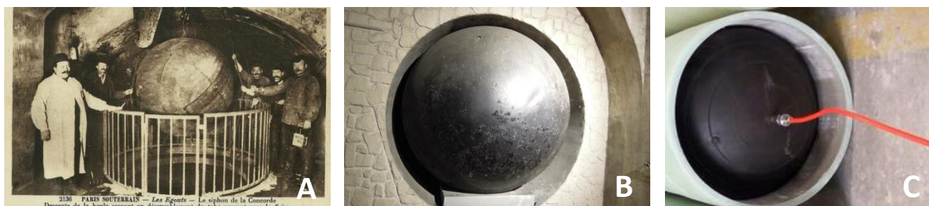
Figure 2. A+B Iron ball to clean Paris’ sewers [Paris Sewer Museum, source: atlasobscura.com (direct link)]. C Rubber water stop [source: Zaoqiang Dacheng Rubber ]
