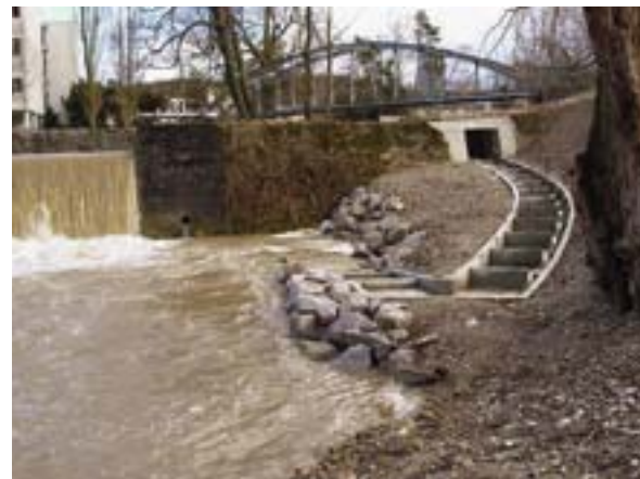
Among the measures recommended in the 10-point plan is the fish-friendly design of hydropower facilities, including fish ladders at dams.
