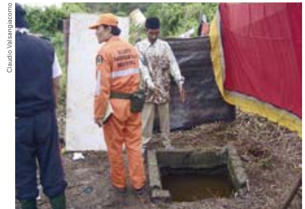
Should this damaged drinking water well in Aceh (Indonesia) be repaired? The well is continuously contaminated by a pit latrine situated behind the black plastic sheet.
