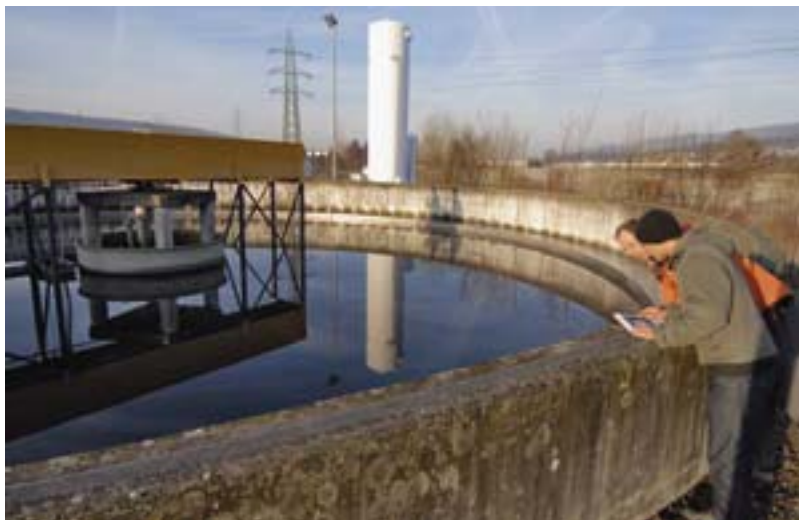
Clarifier at the WWTP Regensdorf. The tank containing liquid oxygen for ozone production can be seen in the background.
