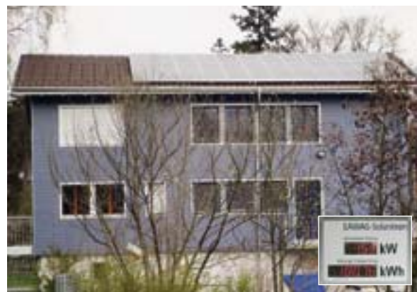
The photovoltaic system on the renovated boathouse in Kastanienbaum has already generated more than 10,000 kWh of power. It was financed by internal CO 2 levies on air travel.
