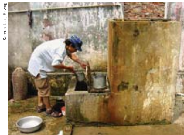
Sand filter for iron and arsenic removal, used by rural households in the Red River Delta (Vietnam).
