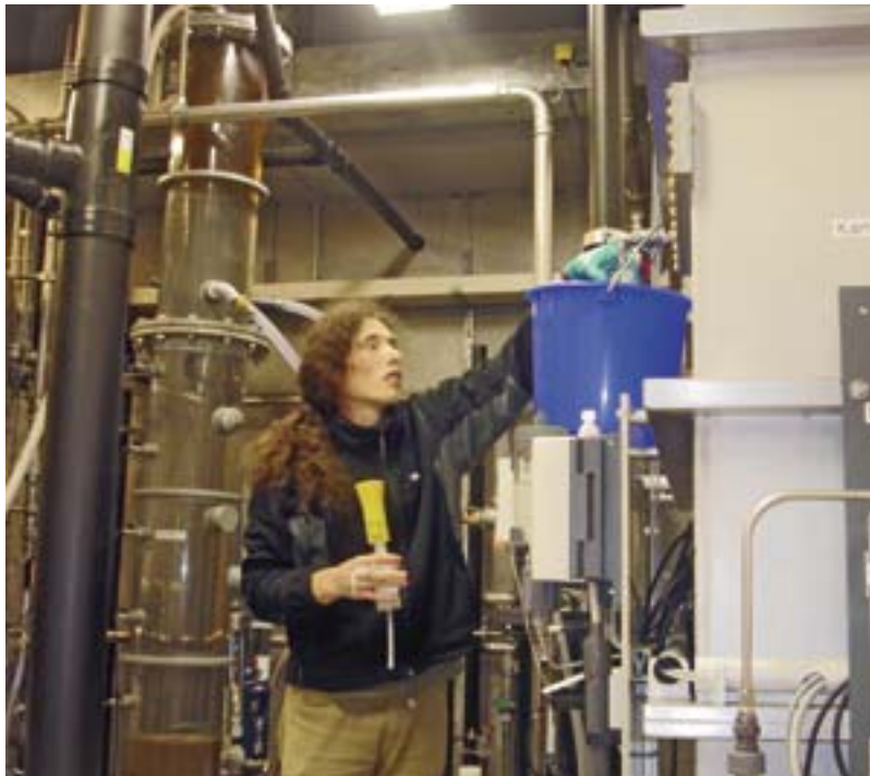
Collecting samples from the ozone reactor in the Wave21 pilot plant at the Lengg lake water treatment facility operated by Zurich's water utility.
