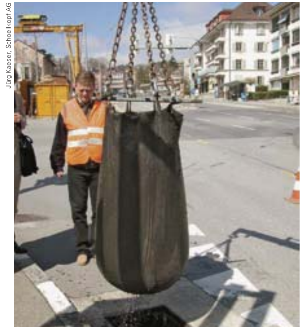
Changing a textile filter bag filled with road sludge.
