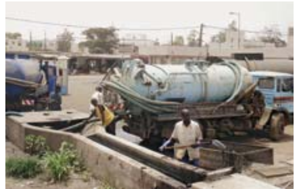
Sludge is delivered to one of the two ONAS facilities.
