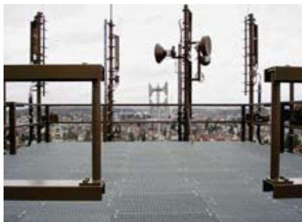
Directional antennas transmit mobile phone signals over the rooftops of Zurich.
