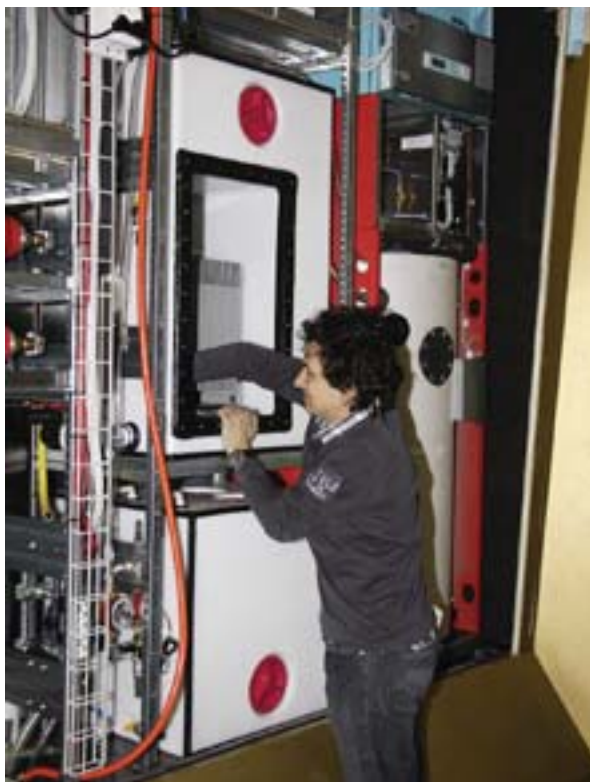
Left: A compact treatment system is installed above the grey water tank in the equipment compartment of “Self”. Centre: Membrane module for preparation of drinking water from roof rainwater. Right: Membrane module for recycling of grey water.
