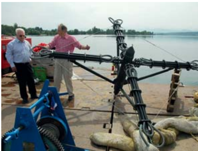
Assembly of the diffusion system which is to supply Lake Greifen with oxygen.
