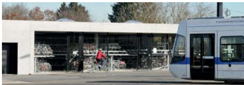
The lockable bike shelter at Stettbach station.
