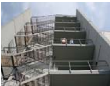
No ivory tower: the renovated laboratory building at Dübendorf.
