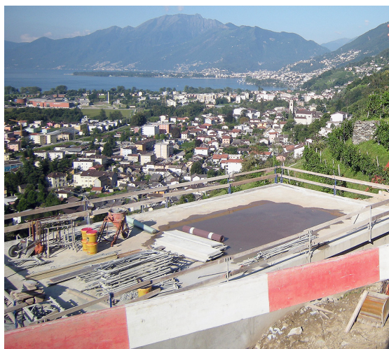
The construction site of the new reservoir, where a drinking water power plant is also being installed.
