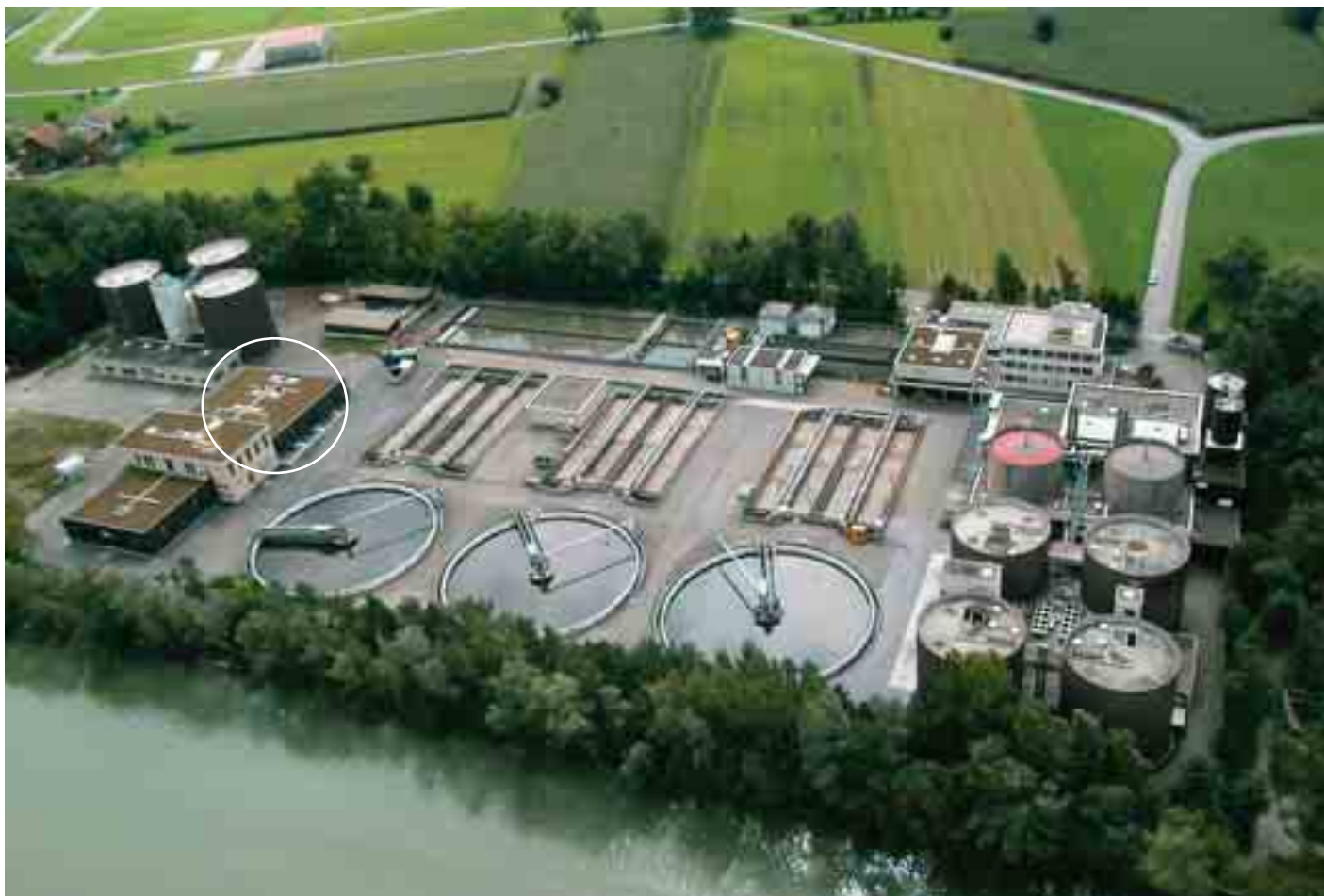
Bird's eye view of the sewage plant Altenrhein: the biofilter facility (ringed) requires 8 times less space than the conventional plant with its 3 rectangular activated-sludge and 3 round settling tanks; the plants each handle half of the incoming waste water.
