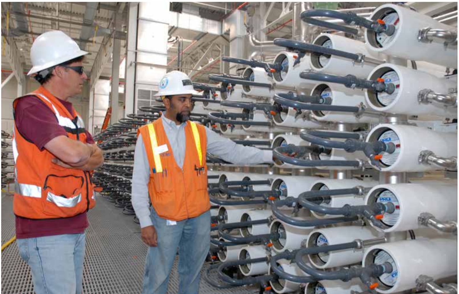
Fig. 1: Potable water reuse has been implemented at the Orange County Water District utility in California. This project, unlike others elsewhere in the state, did not encounter public opposition. Pictured here: the reverse osmosis system.
