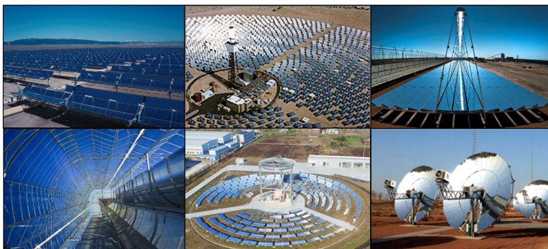
Figure 1. Designs of Concentrated Solar Power plants. Top left: parabolic trough (BLM, 2004); top centre: central tower receiver (Sandia National Laboratories, 2018); top right: linear Fresnel (Laird, 2012); bottom left: Enclosed parabolic trough (Glasspoint Solar, 2014); bottom centre: central beam down tower with ground-level receiver (CNSTE, 2017a); bottom right: Parabolic dish with Sterling engine (Coventry and Andraka, 2017).
