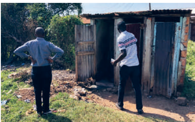
Inspecting shared sanitation facilities in Manyatta, a district in the city of Kisumu, Kenya.
