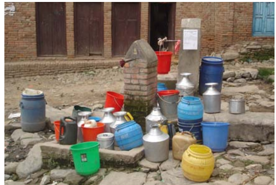
A stand post waiting for water delivery
